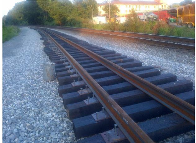
Ties and tie plates have been installed on the bridge and heading south toward the new signals. It won't be long now before the shoofly track will be ready to connect.
