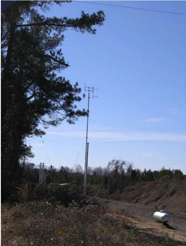
Also is a closer view of antenna. Also you can see the vertical support for the northbound signals in the background, as well as the old signal bridge. The antenna. The two flat looking antennae sticking out to the right, are for the train communications.
